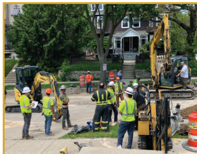
Overseen by the City of Milwaukee Engineering Dept. outstanding work being done by the men from American Construction Services, West Bend and WE Energies as our 2424 W. Kilbourn received new copper replacing old lead line water service
