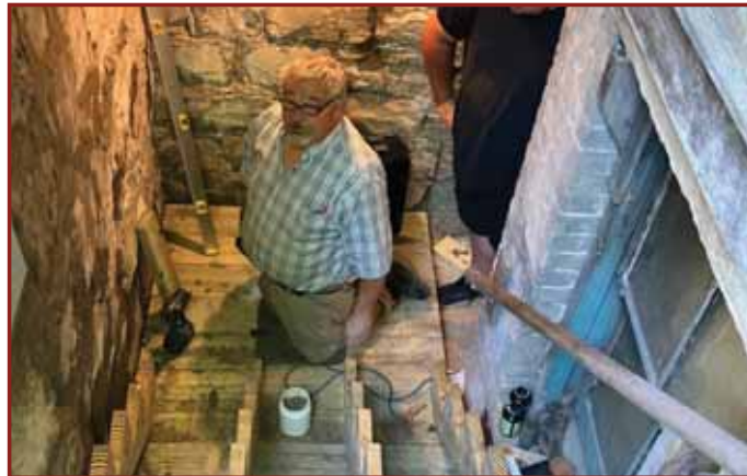
Ranger Kelly carpenter extraordinaire building new steps at 939
